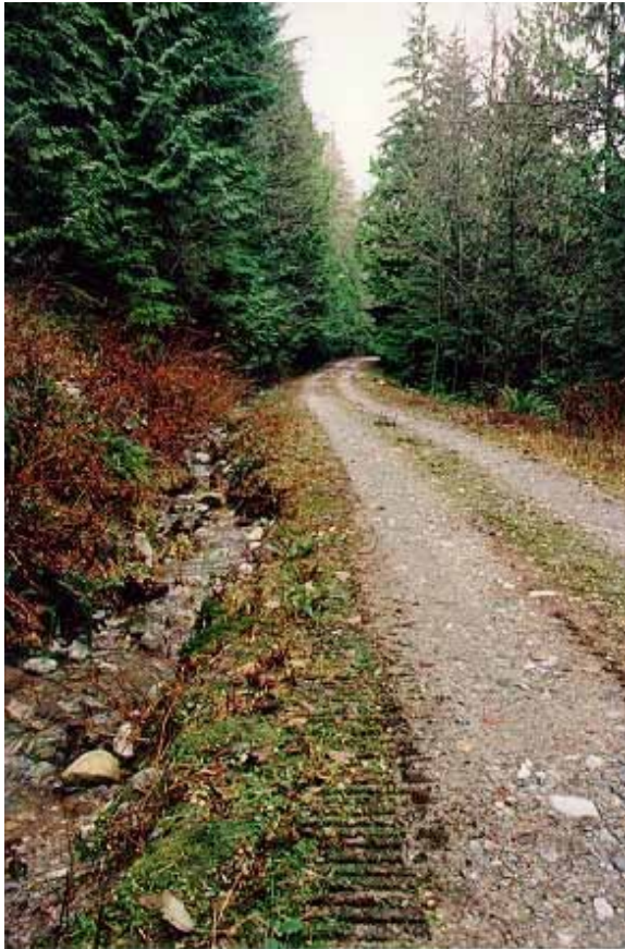
Middle switchback road ditch, looking upslope. Water run-off travels freely for about 300 meters. Old culverts no longer functioning.
