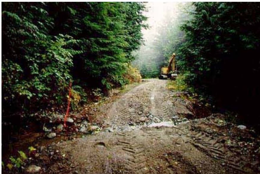
Photo taken November 12, 1995. Excavator on upper Hollyburn road removing old culverts, blocking and digging out ditches. Culvert removed in foreground, and new placement of water bar.
