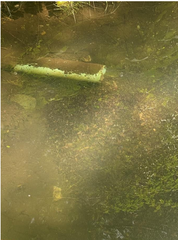
Photo 6. Sediment Build Up on the Water Intake of the Landowner's Water System
