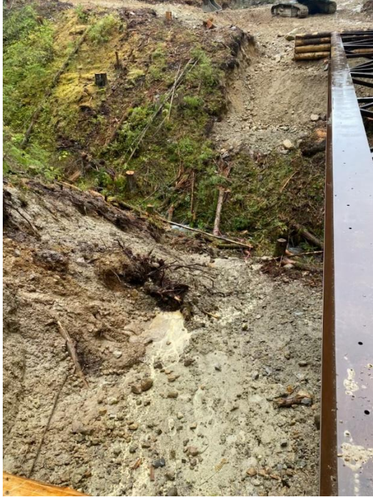
Photo 3. Road Construction Eroding into Roddy Creek November, 2021
