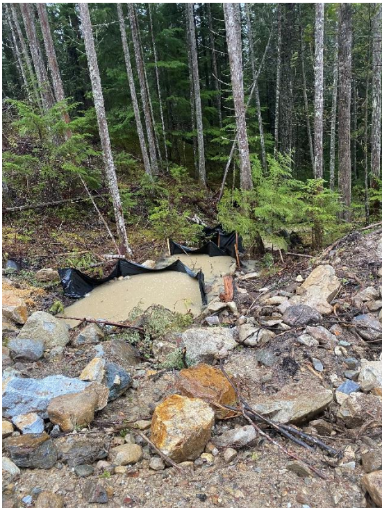
Photo 4. Sediment Control Structures Requiring Maintenance with Extremely Turbid Water, November, 2021
