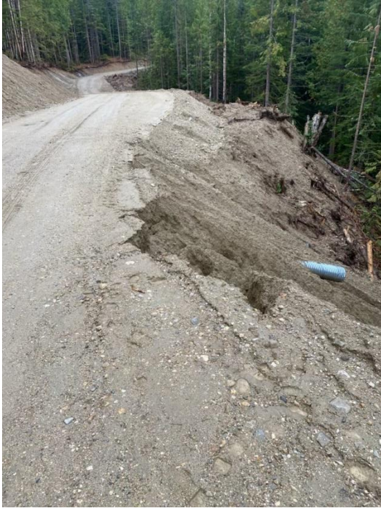
Photo 1. Erosion on Logging Road Above Landowners Water Supply November, 2021
