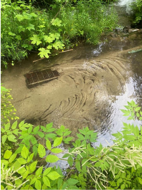
Photo 5. Sediment Build Up in Landowner's Water System Intake
