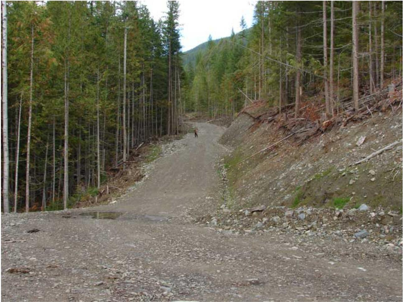
Photos (September 23, 2008) of new road in lower southeast corner of the Arrow Creek Watershed Reserve, above the water intake. The road, cut through kilometers of steep, sensitive glacial soil profiles, will continue to ruin the Arrow Creek, the source of water for the famous Kokanee Beer factory in Creston.
