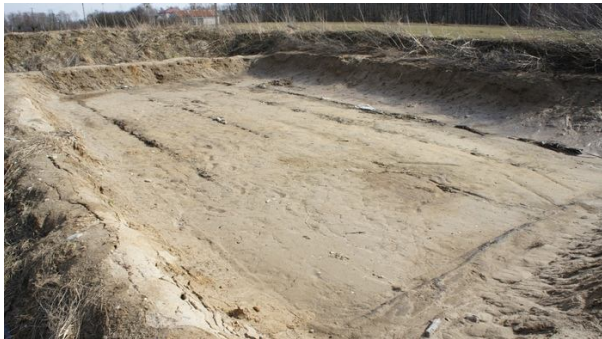
Photos of the area cleared and excavated for drilling fluid and water pits and pad location. In the bottom photo, in the distance, are the stacks of wooden platforms for the fracking pad.
