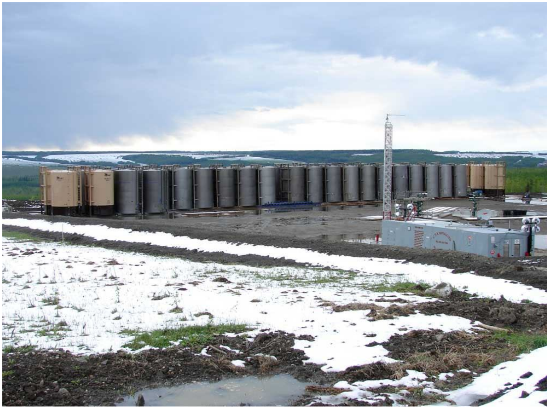
Huge storage tanks for water, with each tank holding a maximum capacity of 64 cubic meters (14,080 imperial gallons), are individually hauled in by trucks and placed on each pad, organized side by side, to be used for the hydraulic fracturing (fracking) procedure.
