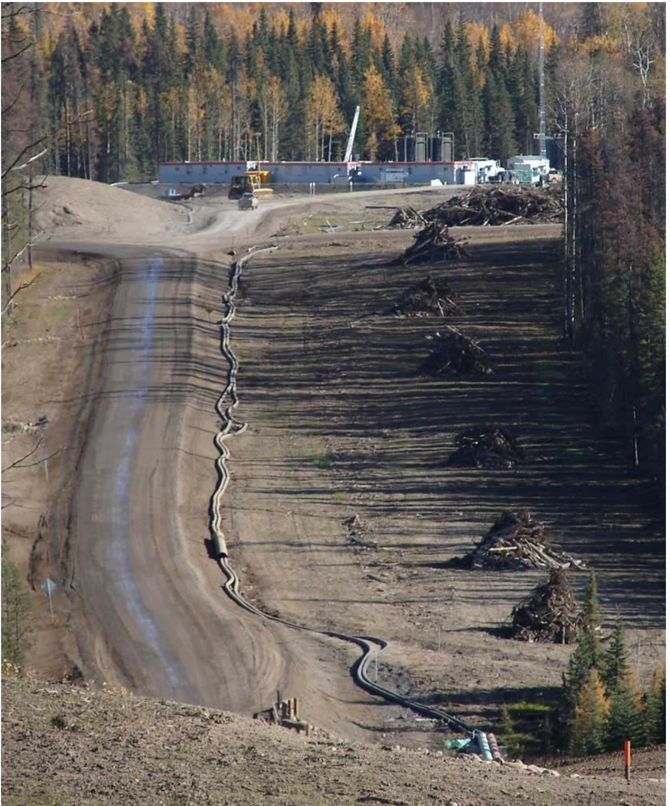
Long lengths of 8-10 inch diameter rubber-like pipes transport the fresh water to fracking sites.
