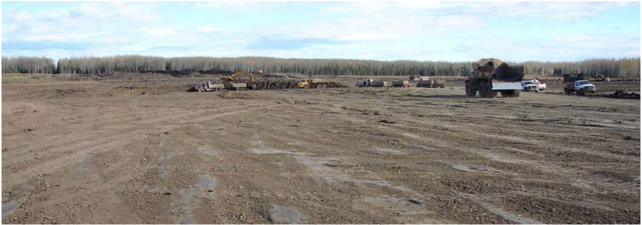
Ground zero at the big Cabin clearing site. (September 29, 2010)
