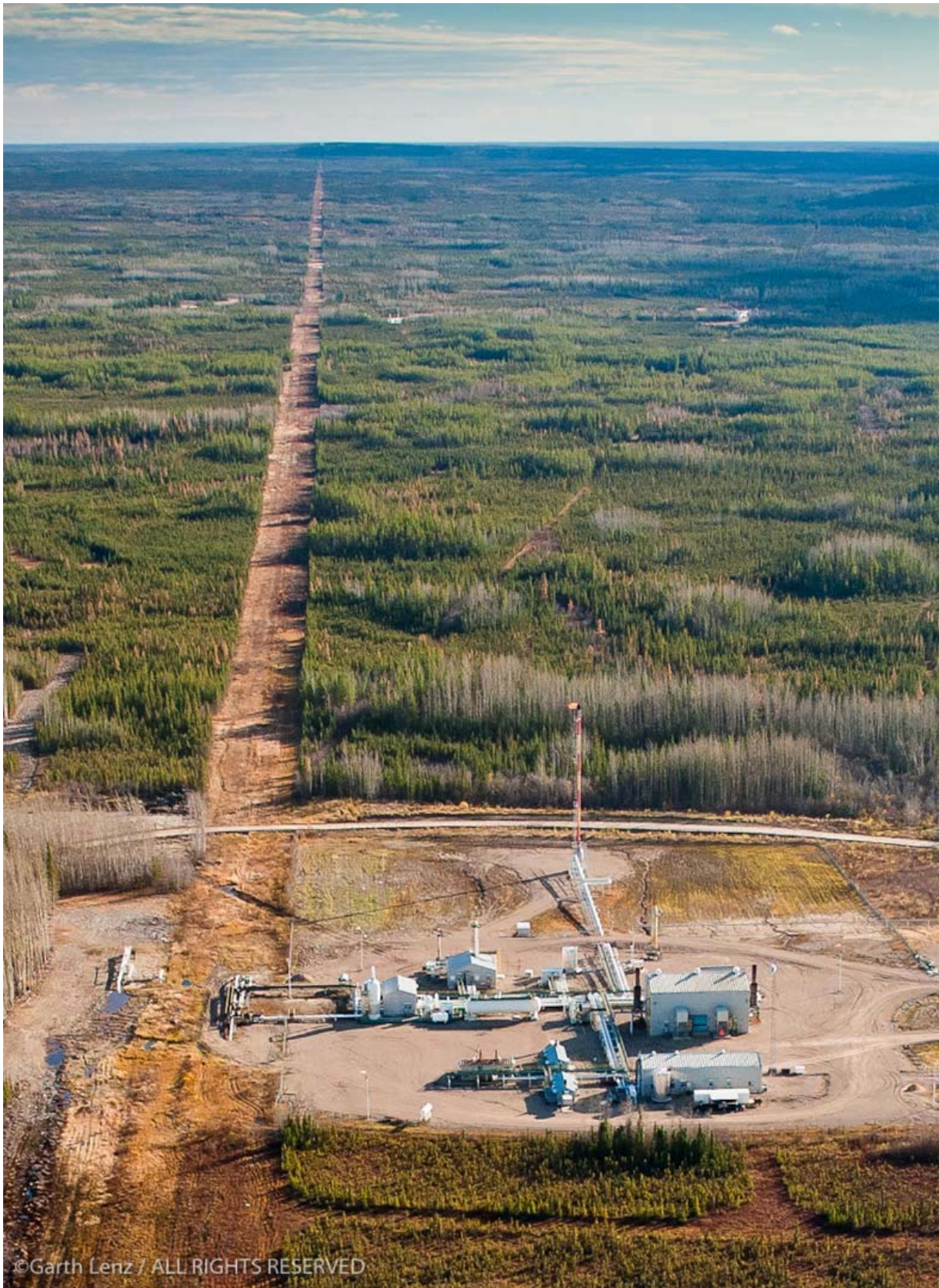
This is Spectra Energy's Cabin Lake Compressor (Booster) Station, B.S. 19. The wide pipeline corridor clearcut which stretches off into the far horizon, is the 25-30 metre wide path of Spectra's 20-inch Louise. (Garth Lenz photo)
