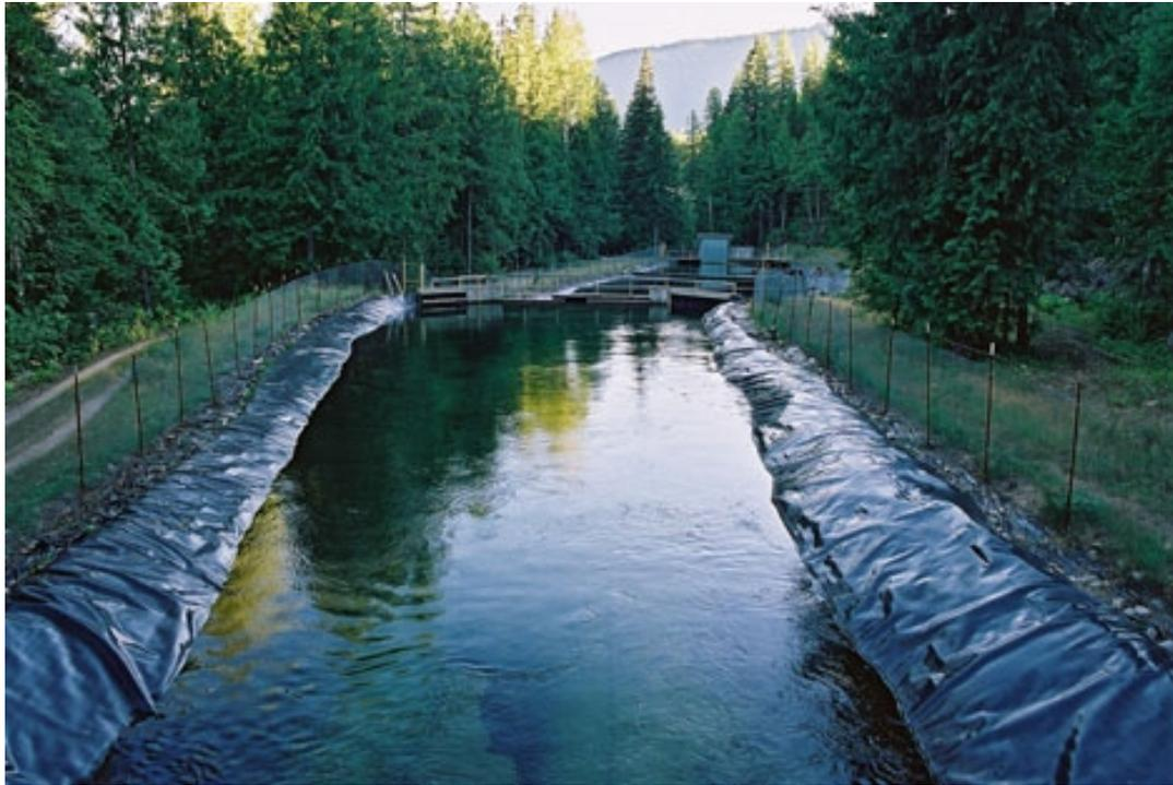
Photo above: Series of two intake settling ponds at Arrow Creek, the water supply for Creston and Erickson. The settling ponds have been here for decades. The new controversial plan for (\$10 million plus) membrane filtration is to pipe the water from this point down to a lower elevation, and then with a series of 16 pumps to pump water to the communities, bypassing the "free" system of gravity used since 1929. (Photo taken August 2000)
