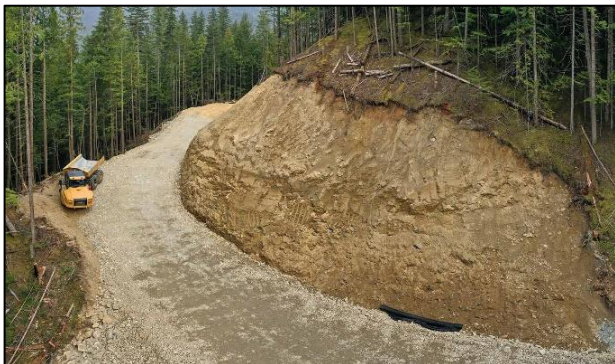
Below, left: same area, September 11, 2022, with new, deep-filled road, showing exposed, fragile clay-silt, vertical bank and very steep cut-slope, above Roddy Creek. Below, right: Same area, September 15, 2022, looking north, with Nels at bottom of vertical cut-slope, showing scale, and Roddy Creek behind Nels.
