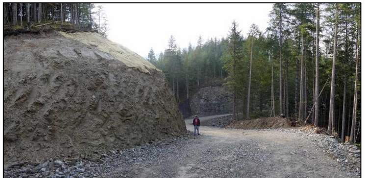
Below, left: same area, September 11, 2022, with new, deep-filled road, showing exposed, fragile clay-silt, vertical bank and very steep cut-slope, above Roddy Creek. Below, right: Same area, September 15, 2022, looking north, with Nels at bottom of vertical cut-slope, showing scale, and Roddy Creek behind Nels.
