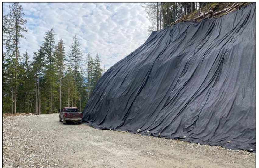
Right: unique cloak mitigation of now troublesome cut-slope above Roddy Creek, September 29, 2022. How much did this mitigation cost? How long will it be effective? How often will it leak, collapse under gravitational pressure, and pollute Roddy Creek?
