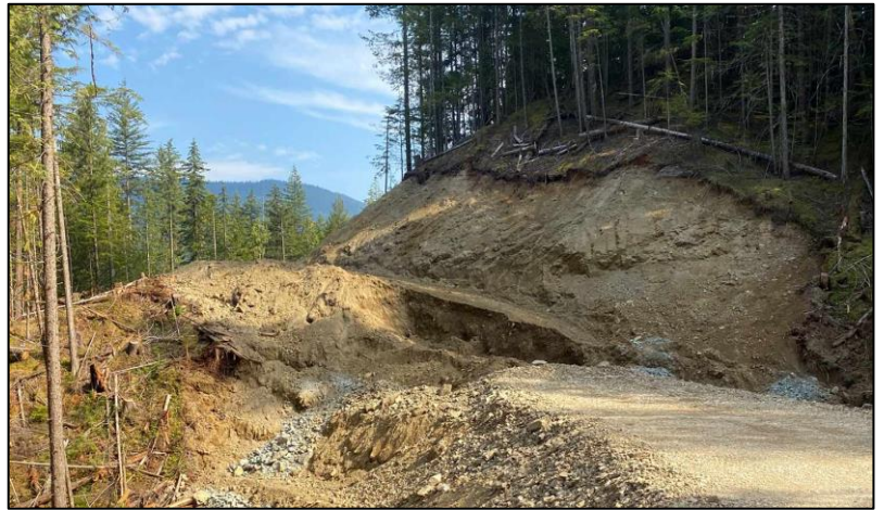
Below, left: same area, September 11, 2022, with new, deep-filled road, showing exposed, fragile clay-silt, vertical bank and very steep cut-slope, above Roddy Creek. Below, right: Same area, September 15, 2022, looking north, with Nels at bottom of vertical cut-slope, showing scale, and Roddy Creek behind Nels.
