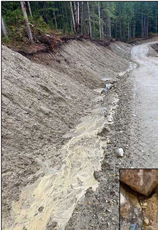
Right: partially blocked culvert on northern section of Roddy FSR, and erosion of downslope prism of Roddy FSR, September 6, 2021.
