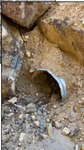
Right: partially blocked culvert on northern section of Roddy FSR, and erosion of downslope prism of Roddy FSR, September 6, 2021.
